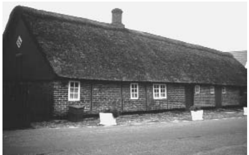
Fig. 4.7 : Timber-framed house from Nordby on the island of Fanø. It dates from the eighteenth century and represents the time before brick-building became dominant. Photo: S. Søndergaard
