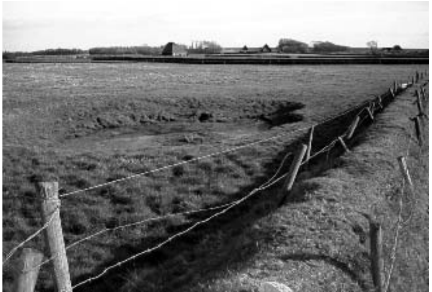
Fig. 2.18: Tuunwallen on Texel, The Netherlands Photo: D. Marrewijk
